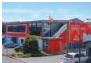
Fujitsu General New Zealand Ltd. (Nowa Zelandia)
